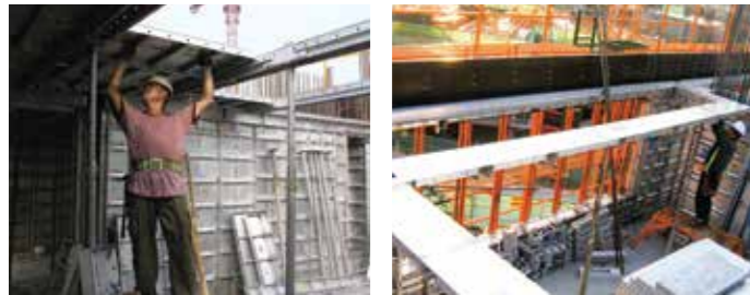
+5 Installation of slab panels
