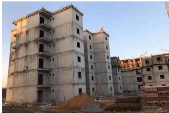
+ 100 logements LPA, Chelf - Algeria - K-Al Form
