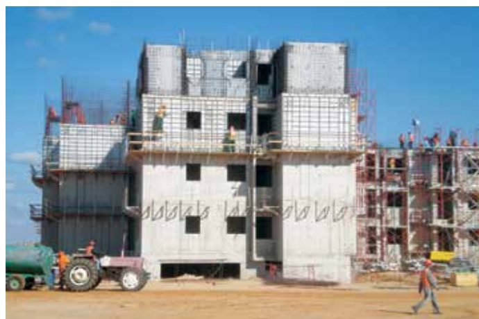
+ 50,000 housing project, Tripoli - Libya - K-Al Form
