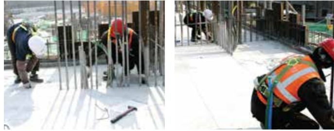
+1 Structural line and level check
