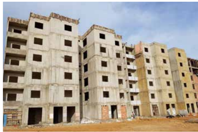
+ 500 logements AADL, Mostaganem - Algeria - K-Al Form
